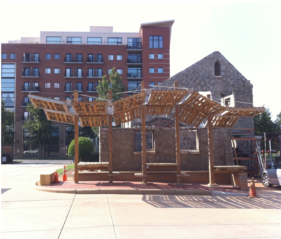
Figure 5- Final constructed canopy nearing completion
